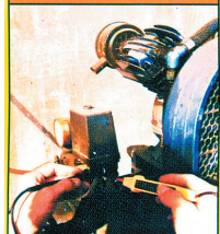
TESTS DC VOLTAGE
